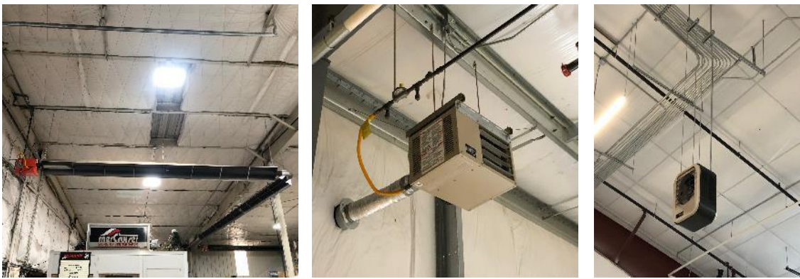
Figure 18: Gas infrared, gas furnace, electric resistance, and ductless mini-split HP, all used freeze protection.
