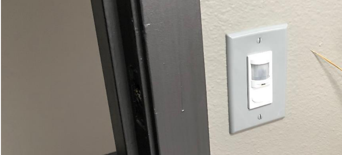
Figure 12: Occupancy control in an office.
