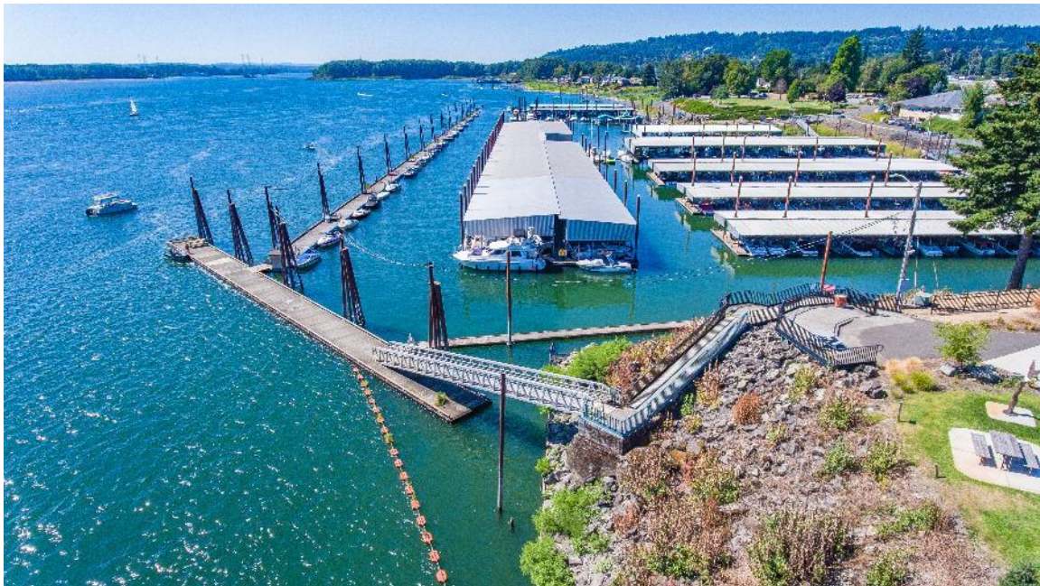
Figure 1: Parker's Landing Marina was established in the early 1950s and includes over 350 moorage slips as well as a public boat launch, boat fueling, a boat repair shop, and a restaurant.
