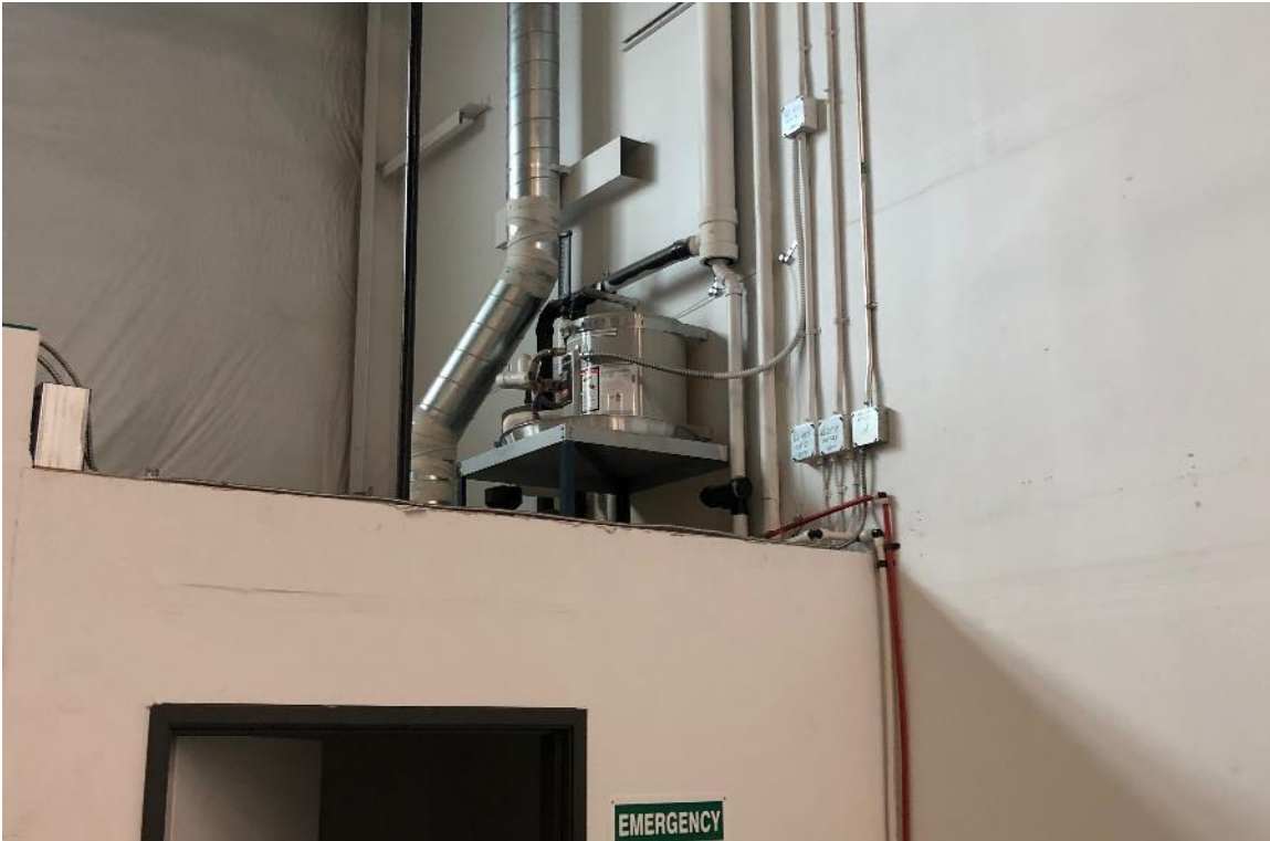
Figure 19: Small water heater serving a single-person lavatory.
