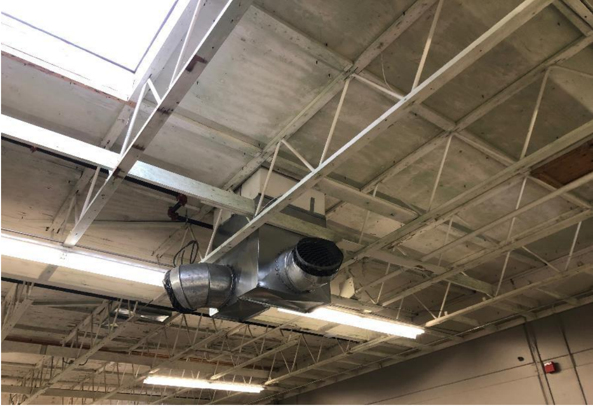
Figure 5: The interior side of a gas-fired RTU in a light industrial building at the Port.
