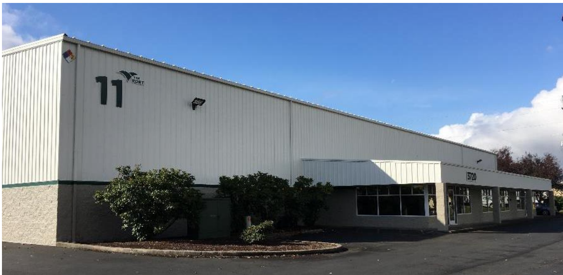
Figure 14: Typical metal building construction of more recent industrial park buildings.
