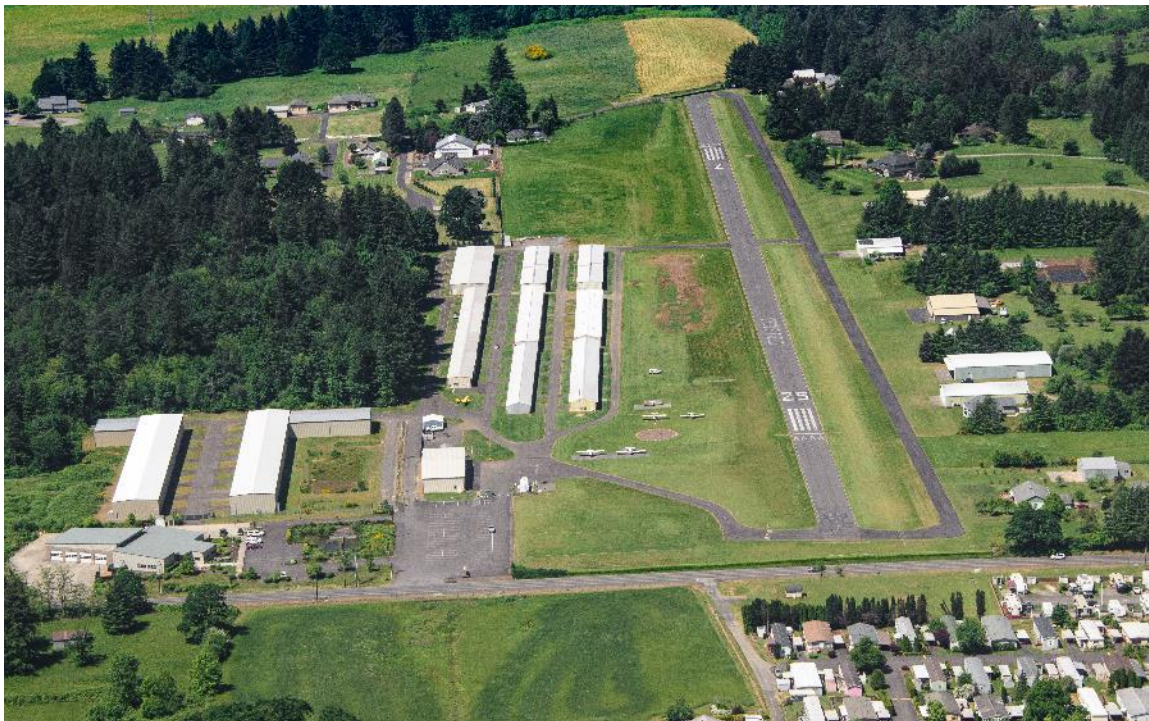
Figure 4: Grove Field is a small airfield with two runways for small aircraft. The airfield includes both storage and commercial hangars.
