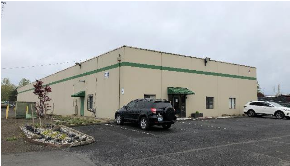
Figure 8: Tilt-up concrete construction like this is typical of some of the oldest generation of light industrial buildings at the Port.
