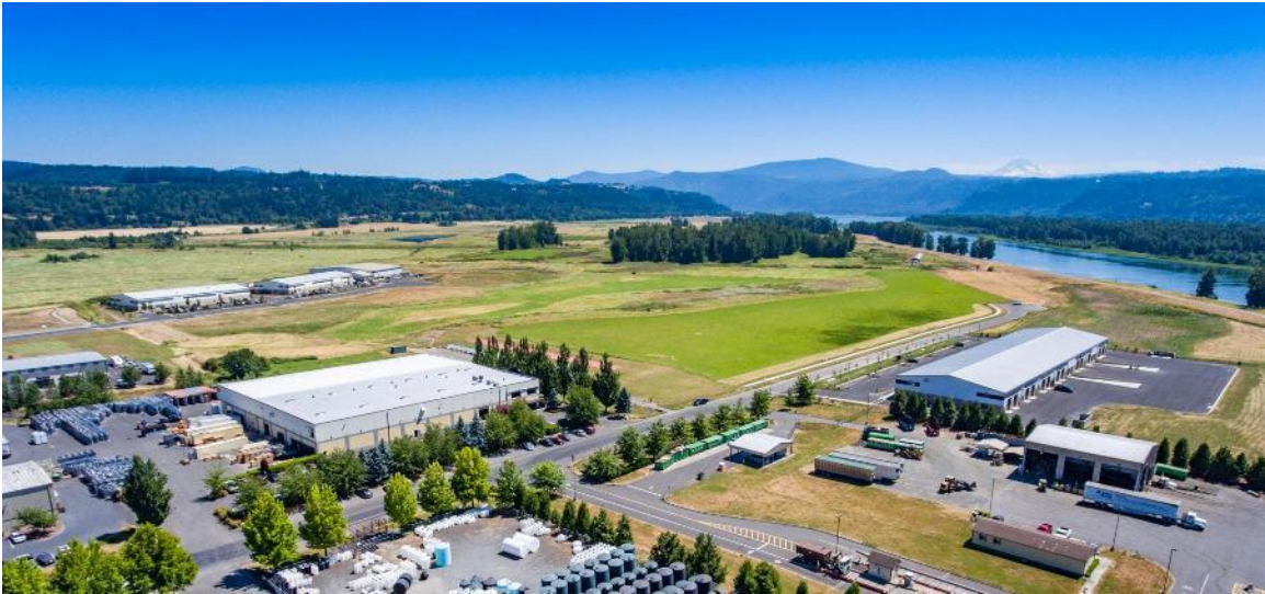
Figure 2: The Industrial Park was created in 1966 when the United States Army Corps of Engineers created a levy along the Columbia. The Park now includes 19, mostly light-industrial buildings with nearly 250,000 sf of total leasable space as well as open parcels
