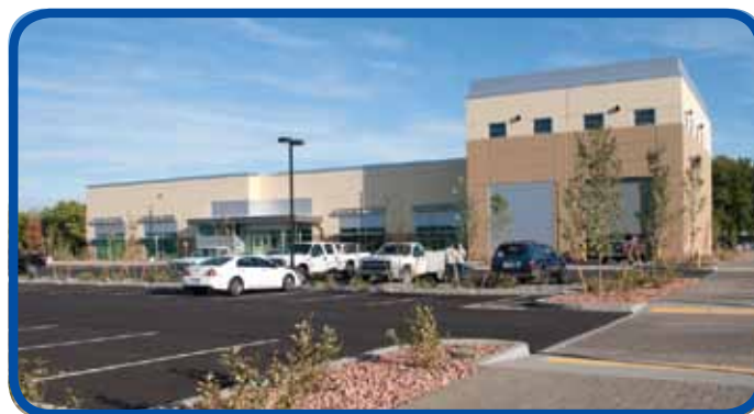
Newly constructed building on the corner of George Washington Way and University Drive.
