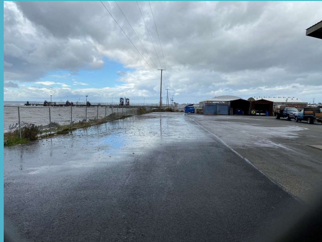
Cornwall Beach – Port Maintenance Facility, Oct 13, 2020
