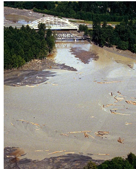
Wikimedia: Toutle River in Flood Stage
