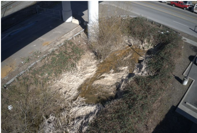
Stormwater Asset Inspections
