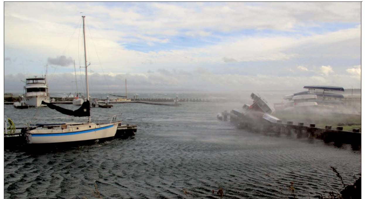
The combination of king tides and winter winds blew through the Point Hudson Marina before the old jetties were replaced, starting in 2022.
