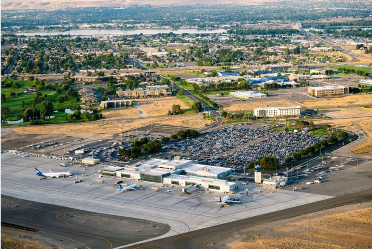
Aerial view of the Tri-Cities Airport, served by five major commercial airlines.
