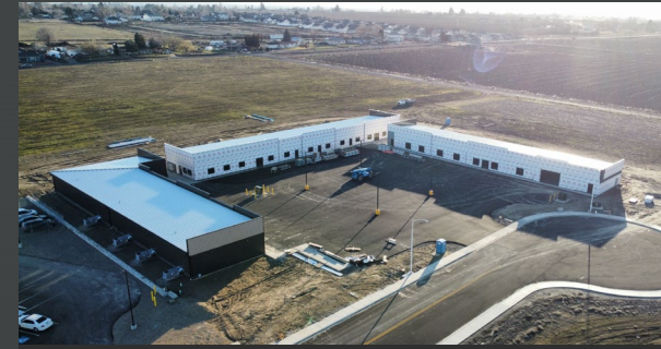
Construction progress ca. March 2025
