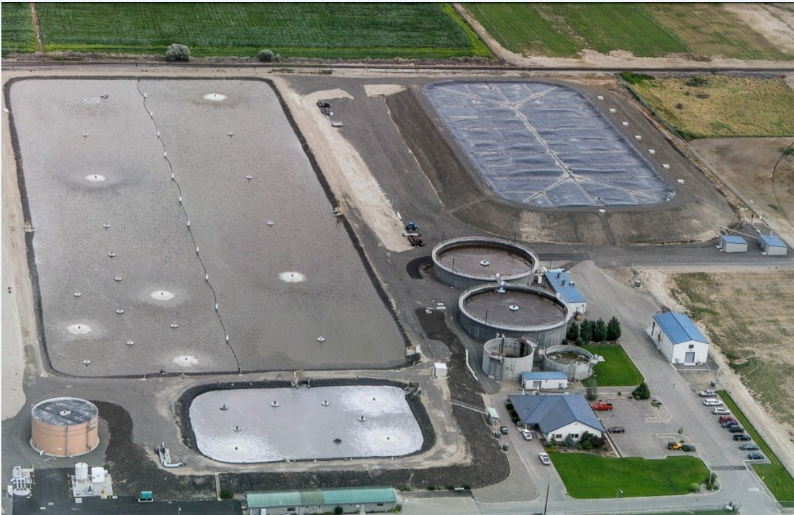
The port's wastewater treatment facility treats food processing waste to irrigate nearby farms, forming a crucial connection in the region's waste reduction and economic development cycle.
