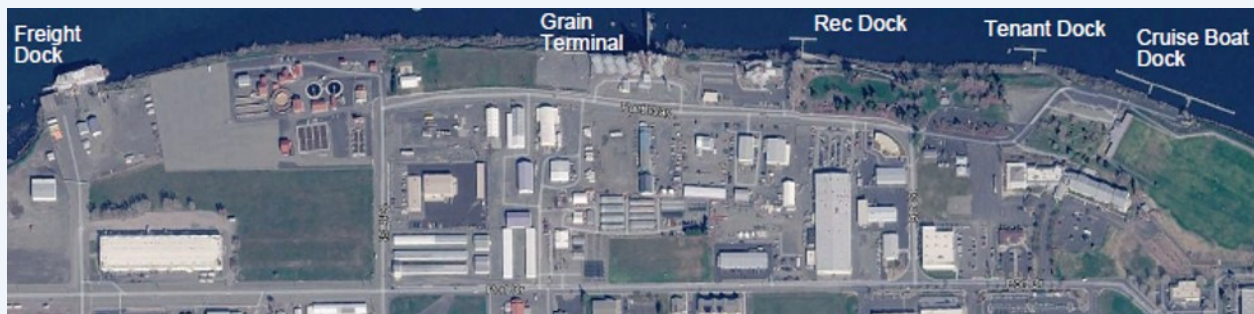
An aerial view of some of the waterfront infrastructure at the Port of Clarkston. Image courtesy of the Port.
