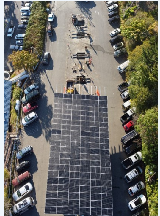
The Port’s solar canopy under construction, as viewed from above. Image courtesy of the Port.
