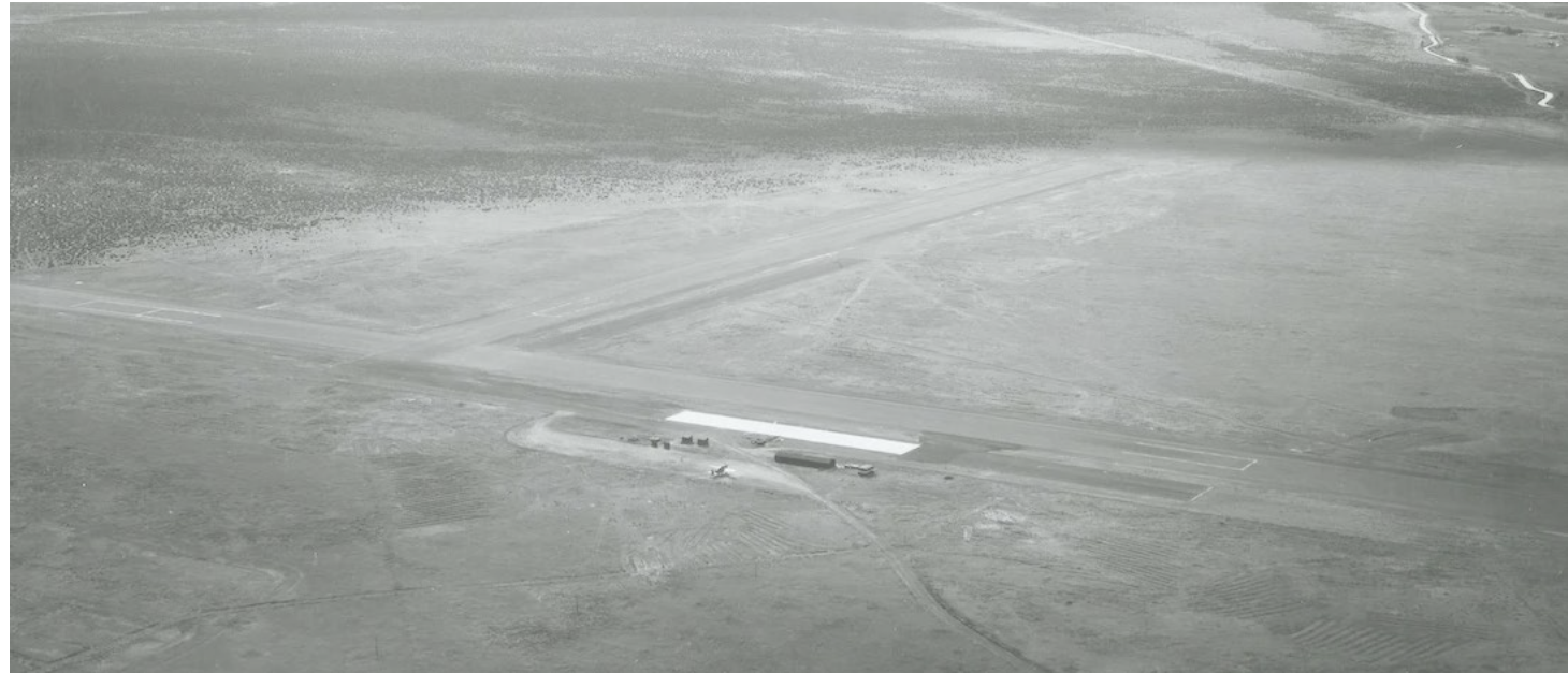
The steel runway at Vista Field for carrier deck landing and catapult takeoff training (center brighter area) on May 26, 1945. Photo courtesy of the National Archives and Records Administration
