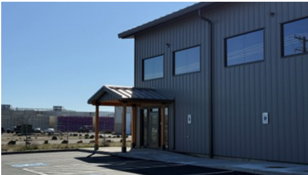
The entrance to Building 153 in Dallesport, home of Columbia Distillery.
